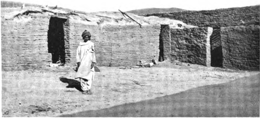
INTERIOR OF REST HOUSE, MUKAK.
